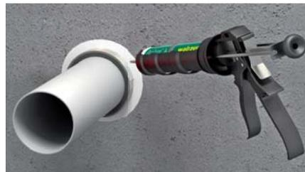
2. Put some mineral wool as backfilling, fill 25 mm in the depth with Acrylic or Silicone Fire Sealant
