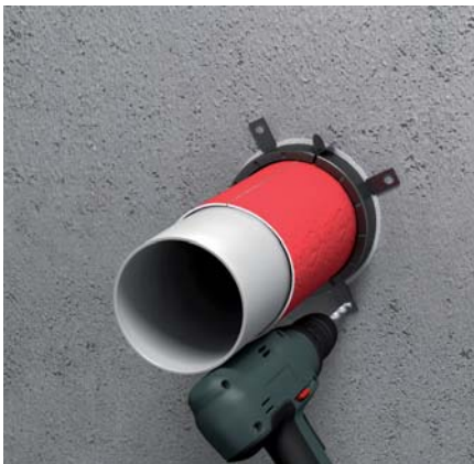
4. Drill (bending and sliding of fixing tabs is permitted)
