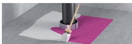
4. Apply Tangit FP 800 Fire Protection Coating on the foam with an overlap of 3 cm on the floor / ceiling
