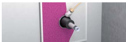
4. Apply Tangit FP 800 Fire Protection Coating on the foam with an overlap of 3 cm on the wall
