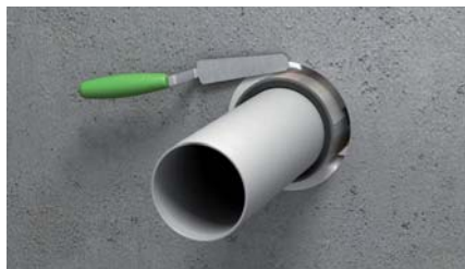
5. Fill the opening with acrylic, foam or mortar
